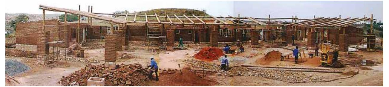
Mud bricks on a concrete block plinth; hollow piers attached and detached support the roof structure of gum-poles.
